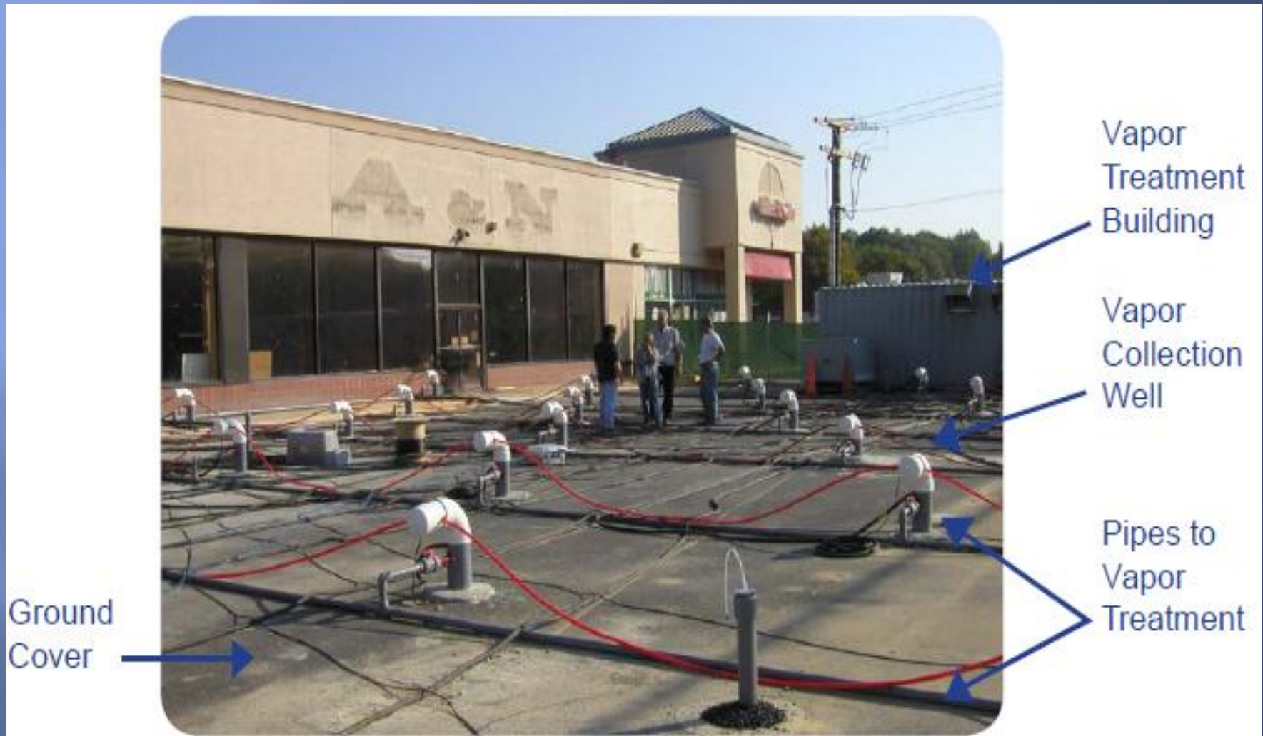
ERH system cleans up contaminated soil and groundwater.
