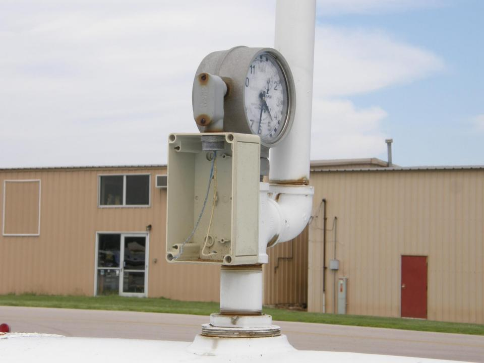
Small diameter piping must Be adequately supported
