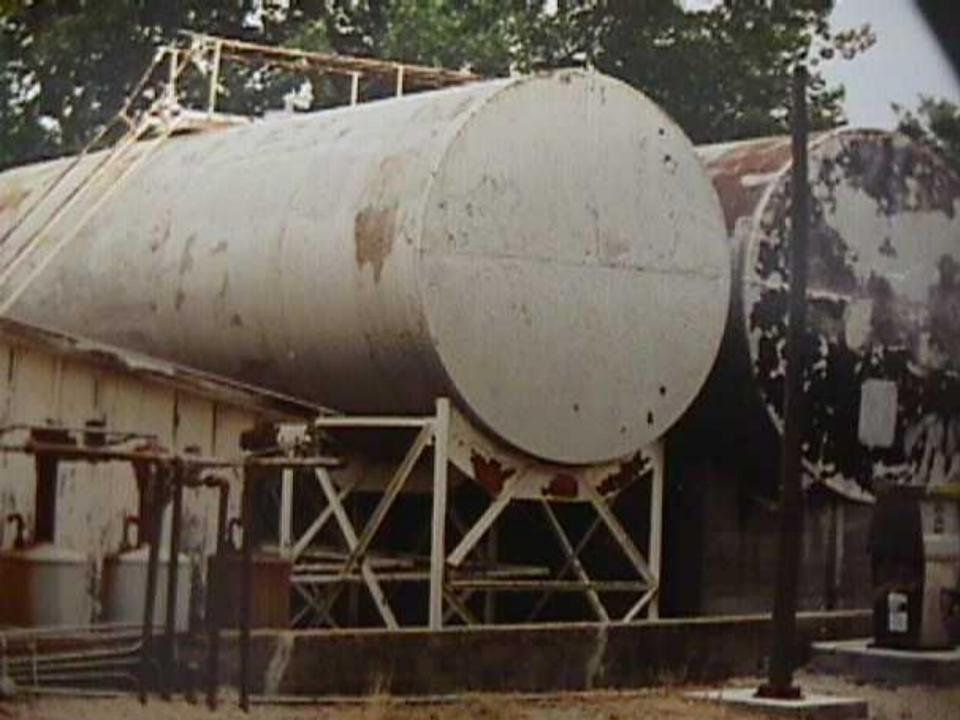
4.4 At service stations where tanks are at an elevation, which produces a gravity head on the dispensing device, the tank outlet shall be equipped with a device, such as a solenoid valve, positioned adjacent to and downstream from the valve specified in the following section (4.5), so installed and adjusted that liquid cannot flow by gravity from the tank in case of piping or hose failure when the dispenser is not in use. (NFPA 30A 1996, 2-1.7)
