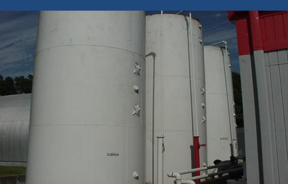
Ozark tank farm featuring the UL 142/58 convertizontal side draft. Very rare 4.7 Tanks storing Class I and Class II liquids at an individual site shall be limited to a maximum individual capacity of 12,000 gallons and an aggregate capacity of 40,000 gallons unless amended by the Director of Agriculture if justification for the need for additional is provided in writing and the level of safety to public and property will not be diminished. (NFPA 30A 1996, 2-4.2.1 & 2 CSR 90-30.050 (13))
