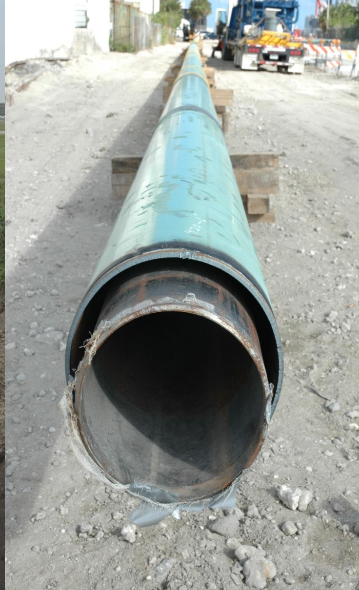
Steel Bulk Product Piping with Secondary Containment - Installation concerns
