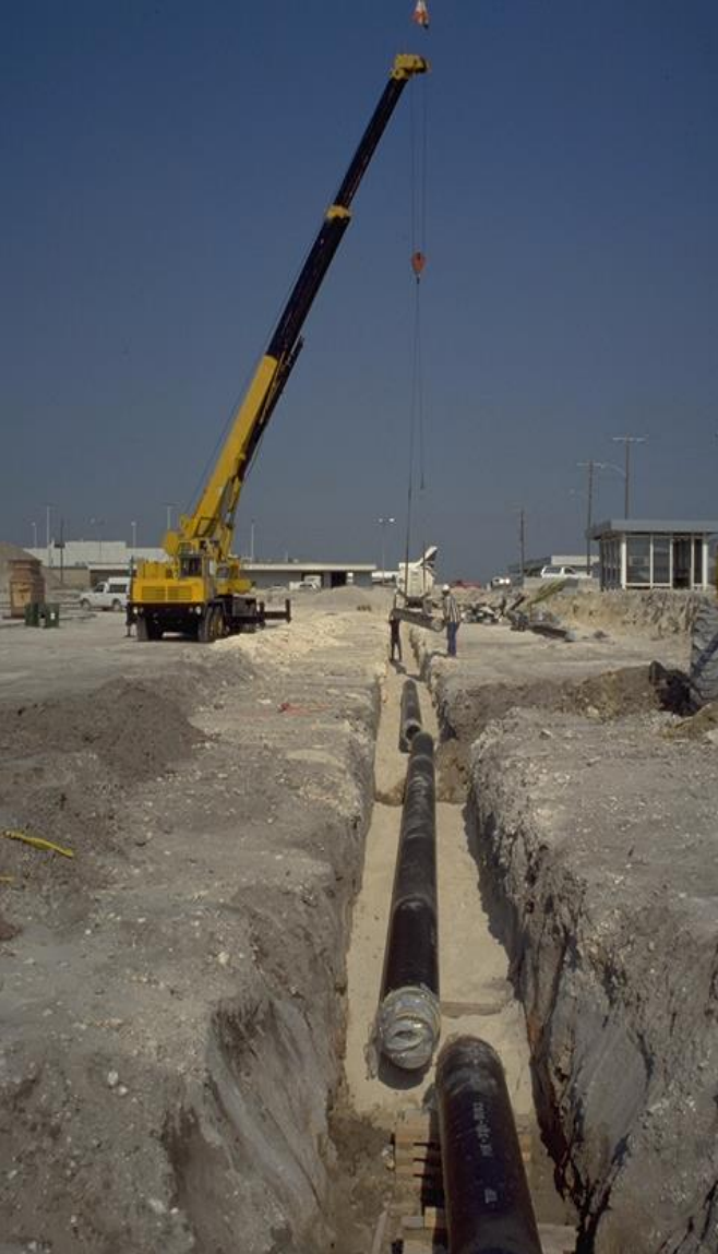
Steel Bulk Product Piping with Secondary Containment - Installation concerns
