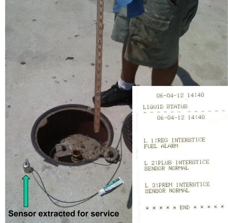
**Double-Wall Piping Leak Detection**
