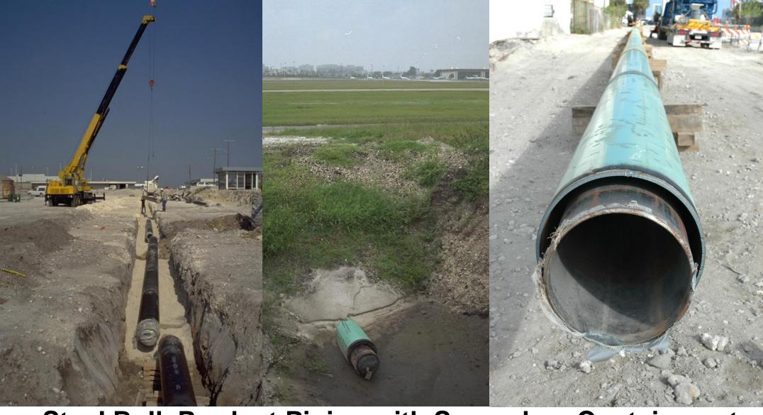
Steel Bulk Product Piping with Secondary Containment
