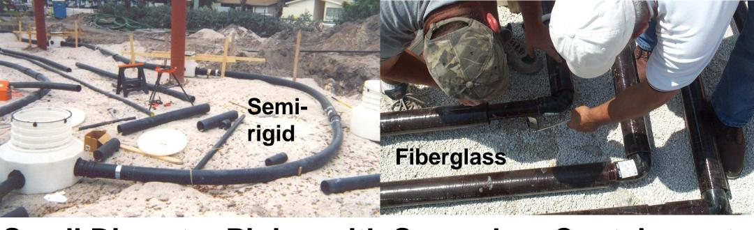
Small Diameter Piping with Secondary Containment
