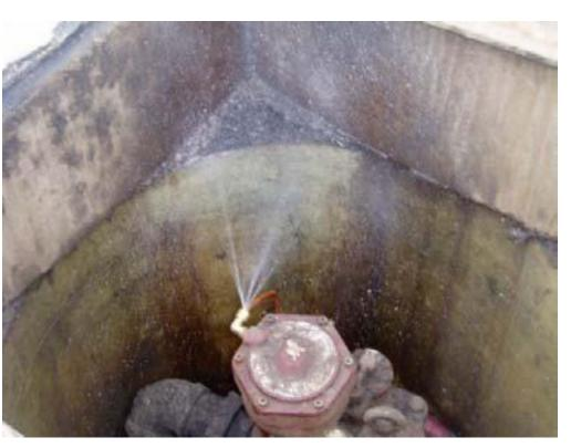
**Leaking Line Leak Detectors**
