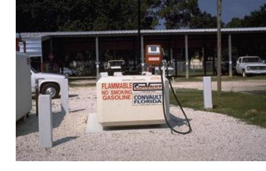
**AST Secondary Containment - Shop-fabricated Tanks**
