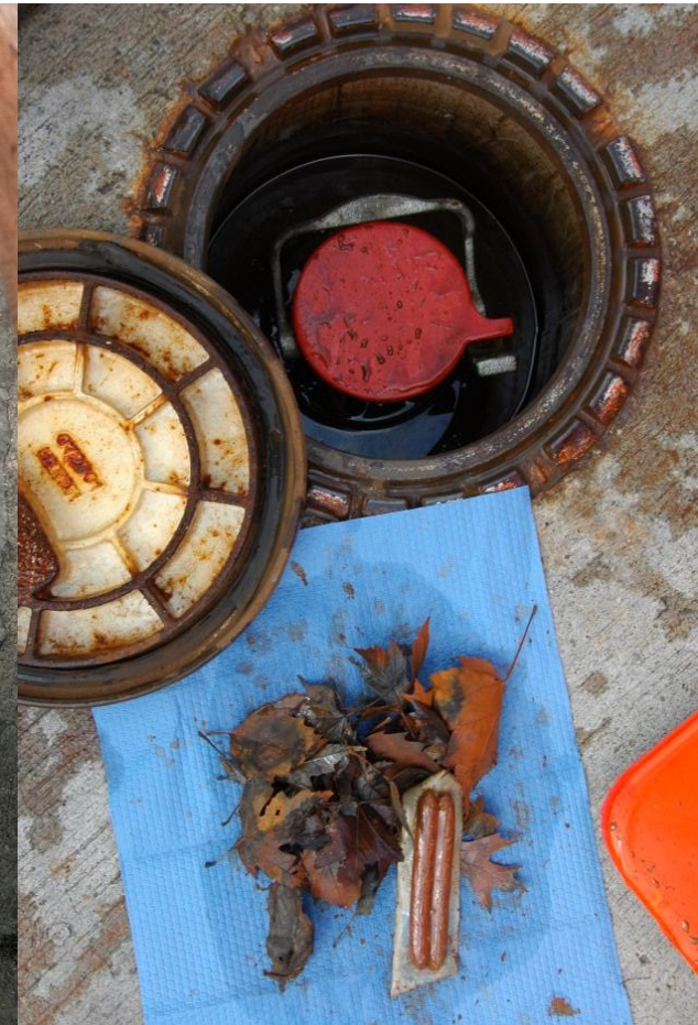
Cleaning debris from sumps
