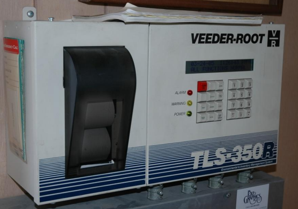
Automatic Tank Gauges
